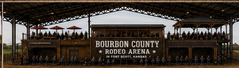
SOUTH END VIEW
